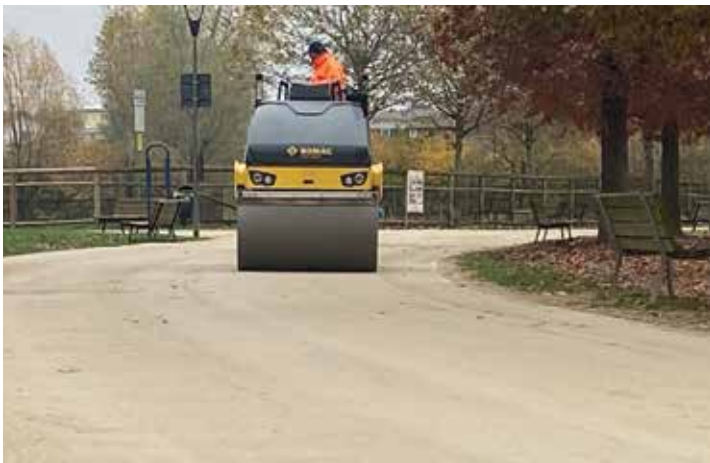
3. | Compaction with a suitable roller
