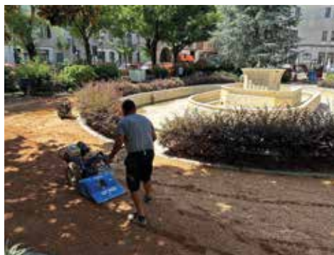
2. | Mixing treated soil with GREEN WAYS® solution
