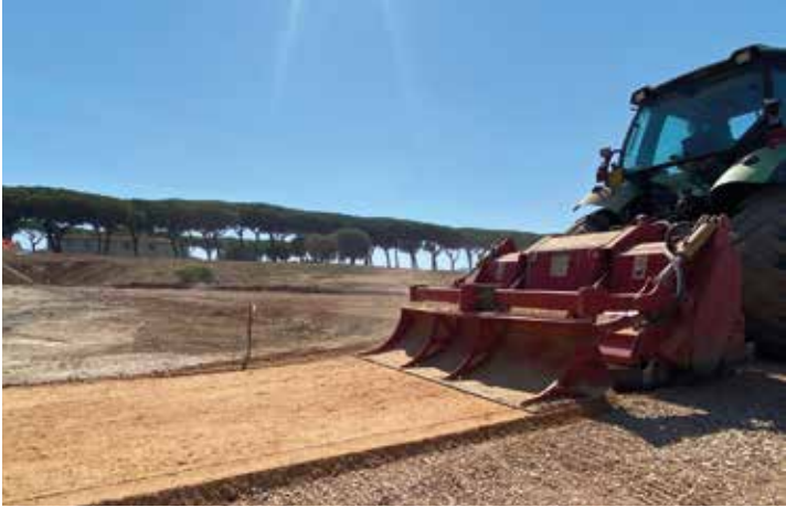
1. | Milling soil present in situ
