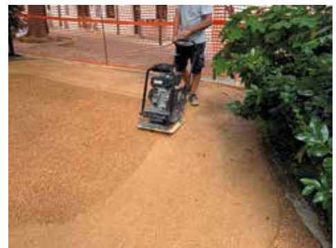
3. | Soil compaction
