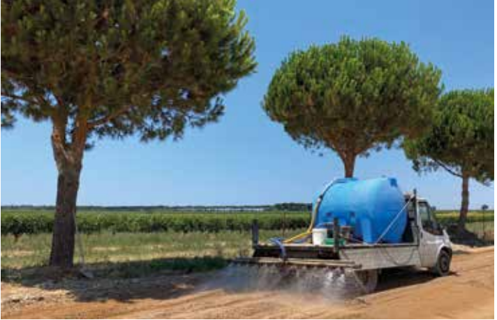
2. | Green Ways® solution sprinkling
