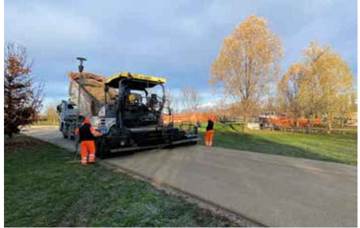
2. | Cold laying of soil treated with Green Ways® solution
