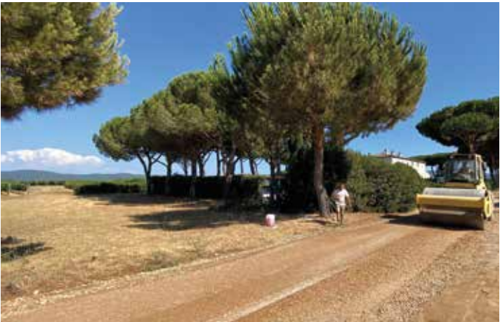
4. | Compaction with a suitable roller
