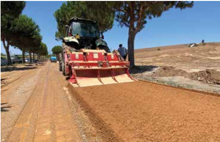
3. | Mixing the treated soil with GREEN WAYS® solution
