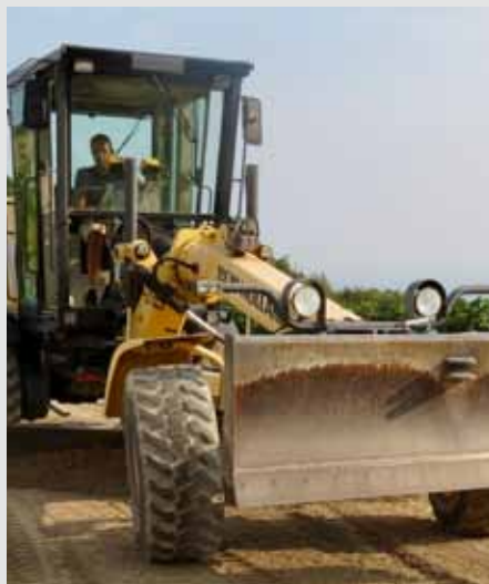
2) Shaped surface with motor grader and subsequent compaction
