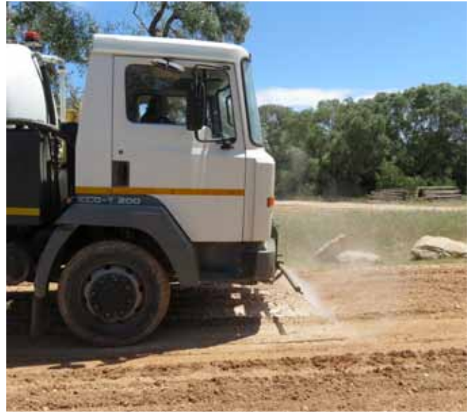
2) Spray stabilizer mixed in water
