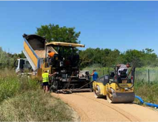
3) Laying of the Soil treated with binder by paver machine and subsequent compaction
