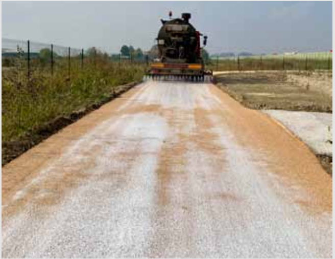
4) Top coating with dust control binder
