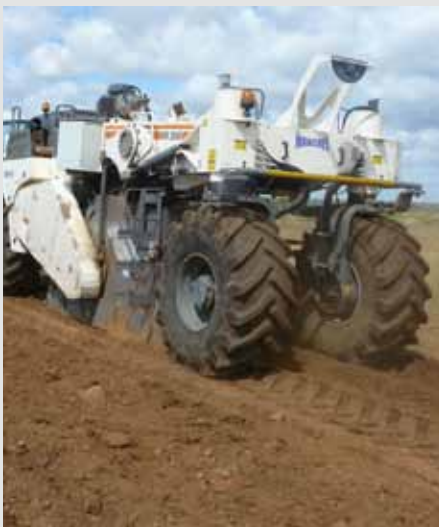
1) Spray stabilizer mixed in water and mixing of the soil
