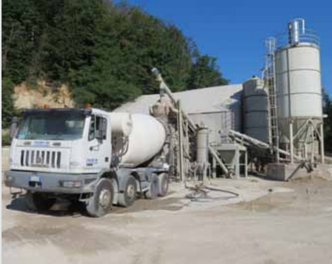
1) Soil mixing with water and binder in a stationary mixing plant or truck mixer
