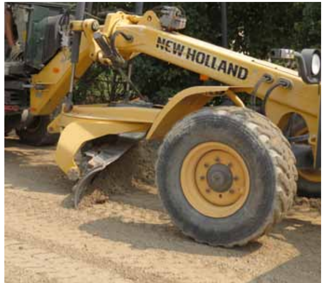
4) Shaped surface with motor grader
