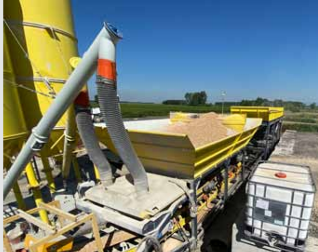
2) Soil mixing with water and binder in a mobile mixing plant
