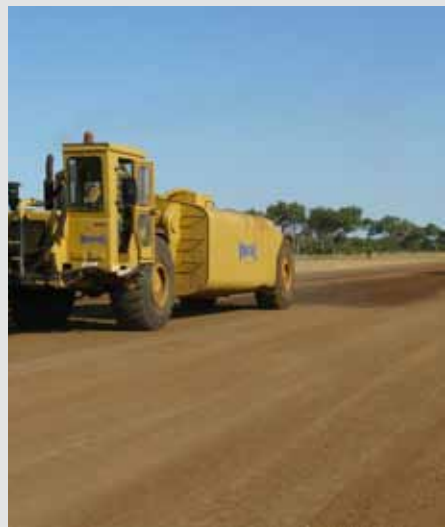
3) Top coating with dust control binder
