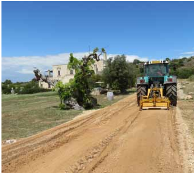
3) Mixing of Soil treated with stabilizer
